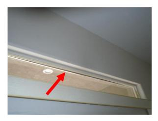
**3.** One screen is missing and screening material at several locations are torn.
