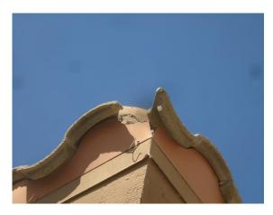
**2.** Several tiles have slid from original position. This can expose the waterproof membrane to solar deterioration.
