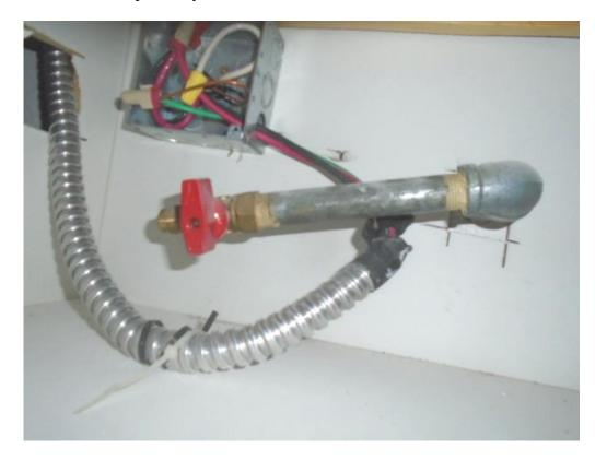
**2.** Outlet located in cabinet at right side of the stove is improperly installed outside its junction box and is at or near contact with combustible material. This is usually a cabinet installer's defect.
