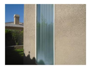
**2.** Displaced seal observed at transom window above slider.
